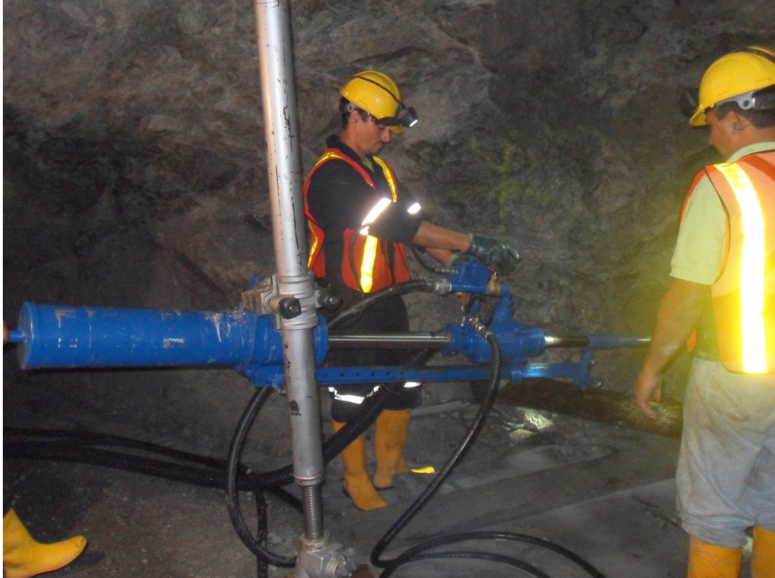
Figure 1: Azuay Project – Underground Drilling
