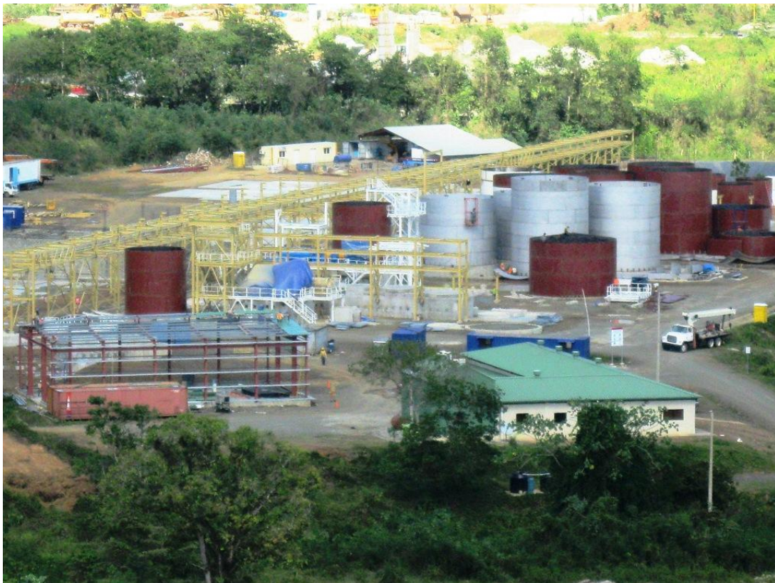
Figure 1: Overview of Construction Site
