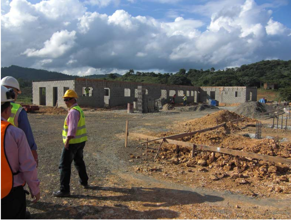
Administration buildings with Workshop foundations in foreground
